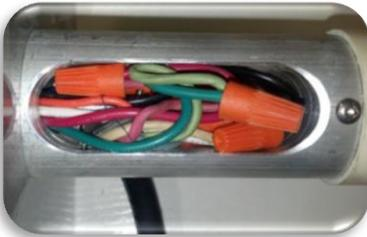
Tuck the wires into the Junction Box. Slide the lid into place and fasten the screw
