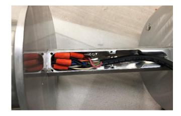
Slide the wire connector/junction cover down the wire and onto the shaft, your cord should be level with the inside of the compression fitting. **Tighten the Compression fitting before setting the cover in place**. Ones you have the compression fitting snug, set the cover into place on the shaft and tighten down with the included 4 screws (Do not overtighten) Wrap up your wire neatly in desired direction.
